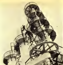
Drying department over an underground natural gas reservoir with a 35,000-million cubic feet capacity.
